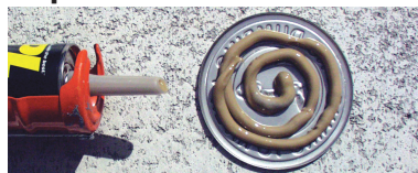
Adhesive Installation on Concrete/Metal Covers
